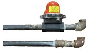
7. Configure new plumbing with PSP valve. Allow 5" to 6" from wall for valve reset shaft clearance.
