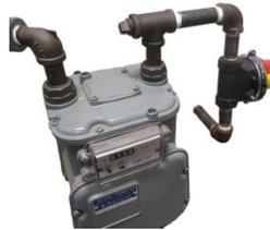
9. Install union gasket and new plumbing from building to meter.
